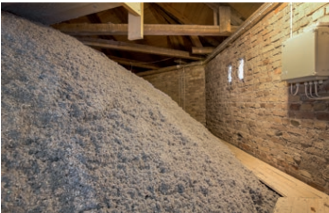
The dome of Beddinge Kyrka was well-packed to keep in the warmth. Right: the church from the outside
