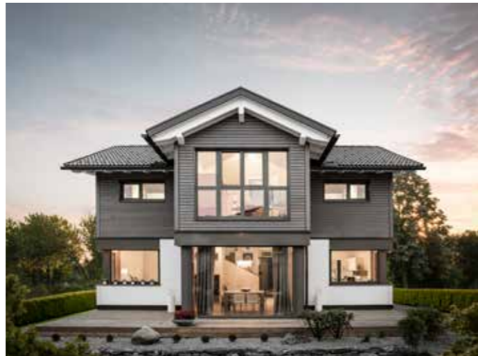
A pre-fabricated house built by Griffner.
