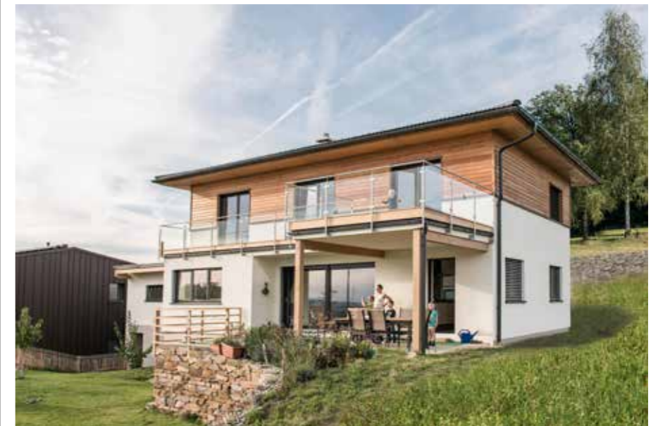
Wolf builds 650 pre-fabricated houses a year.
