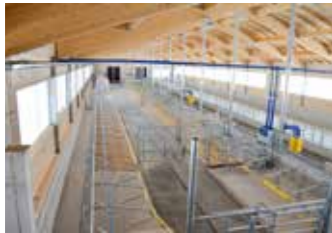
Buildings for agriculture have always been an important part of the company portfolio.
