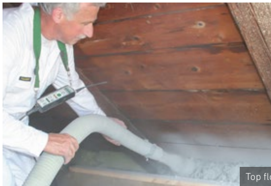
Blown ceiling insulation
