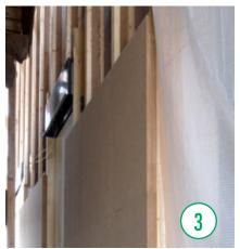
The respective plaster base material is mounted on the perpendicularly aligned spacers. In the case of rear-ventilated facades, a diffusion-open woodbased panel is attached.
