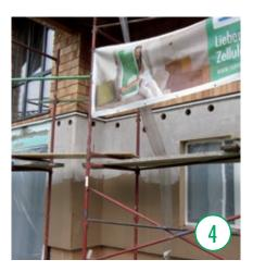
Holes are drilled into the hollow spaces for the injection hose shortly before installing the ISOCELL cellulose insulation.
