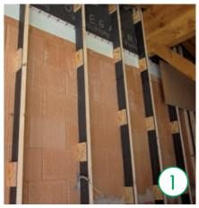
Depending on the thickness of the insulation, timber laths, TJI beams or timber constructions are fastened to the solid wall. The centre-centre distance depends on the requirements of the respectively employed plaster base material.
