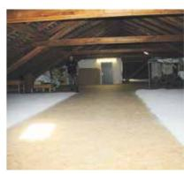
The district of St. Marien chose the WoodyFIX system for the insulation of the attic of its elementary school. Apart from the use of an ecological insulating material — St. Marien is a 'climate protection district' — a deciding factor was that the attic remains usable as an accessible area. With the insulation of the top floor the elementary school in St. Marien now saves 42% heating energy.
