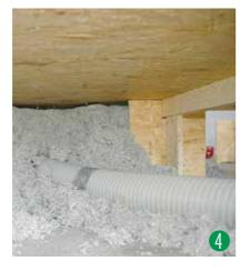
Afterwards the construction is filled with the ISOCELL cellulose.
