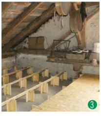
Lay the floor boards and fix them. With an 18 mm OSB wood-based panel, the construction is an accessible system with a very high load capacity.
