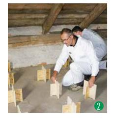
Set up the modules at a centre-centre distance of approx. 80 cm. Then place the 4/6 laths into the cut-outs provided (without screwing).
