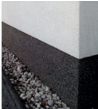
Work carried out according to building standards
