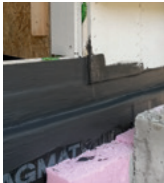
Omega Pobit waterproofs the base of the building
