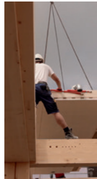
A building with eight floors supported by a solid wood glulam structure.
