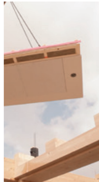
In July 2014 construction works began on K8, KAMPA's new company headquarters.
