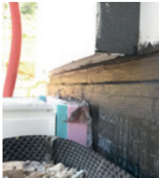
Liquid base waterproofing membranes are capable making even the most complex transitions watertight
