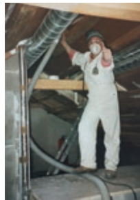
Archive images with the motto "Back then we were already good; today we're even more innovative": ISOCELLERS blowing in cellulose
