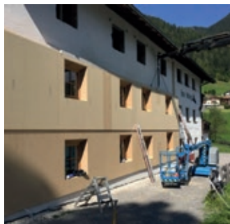
Installing the façade
