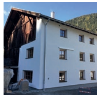
The finished façade
