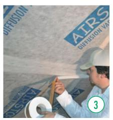
The airtight taping and sealing of overlaps, connections and penetrations is very important. See the brochure 'Air-tightness in detail' regarding this.
