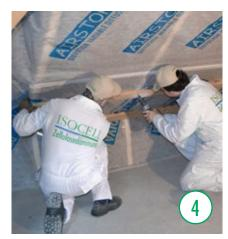
Now the laths are attached at a centre-centre distance of approx. 30 cm. The laths are positioned directly on the sealing of the overlaps in order to additionally relieve the adhesive joints.
