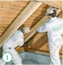
Depending on the desired insulation thickness, the rafters are doubled on the inside of the attic. Two variations are shown here for the construction (see detail drawings).
