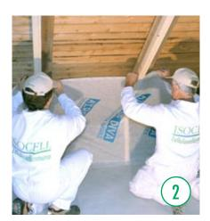
The vapour retarder is laid overlapping and is mechanically fixed by means of tacker staples.
