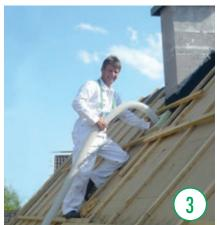
After completion of the sub-roof the cellulose insulation is installed. Within the cavity the fibres become matted to form a compact, seamless insulation mat.
