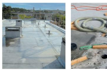
It is so straightforward to make a well-insulated building out of an energy waster. The roofing contractor opened the roof in various places. The company LKI from Nidda-Harb insulated the 600  $m^2$  roof area with 30 cm ISOCELL in just a short time.
