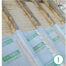
The old roof cladding is removed. The vapour barrier (e.g. FH FORTE) is laid above the rafters in so-called sub-top procedure and fixed at the side with laths or press-on strips. Airtight sealing is achieved with the AIRSTOP adhesive system.
