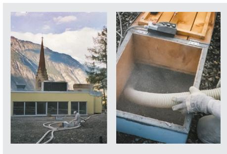
On many old residential buildings the upper ceilings of concrete are below a slightly sloping wooden construction as roof. Or these are so-called 'ERTEX roofs' in concrete. High loss of heat in winter and rapid heating-up in summer are inevitable.
