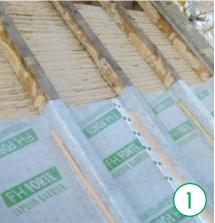
The old roof cladding is removed. The vapour barrier (e.g. FH FORTE) is laid above the rafters in so-called sub-top procedure and fixed at the side with laths or press-on strips. Airtight sealing is achieved with the AIRSTOP adhesive system.
