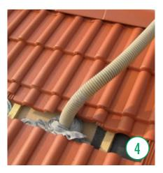
On previously tiled roofs only a few tiles need to be removed to make room for installation work.
