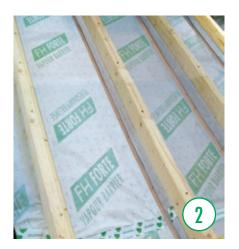
Old battens often do not provide enough space for today's insulation standards. In order to allow for the insulation thickness the battens are doubled.
