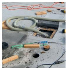
It is so straightforward to make a well-insulated building out of an energy waster. The roofing contractor opened the roof in various places. The company LKI from Nidda-Harb insulated the  $600 \, \text{m}^2$  roof area with  $30 \, \text{cm}$  ISOCELL in just a short time.
