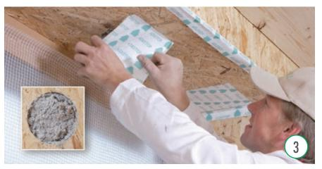
The cellulose is installed in the hollow spaces by means of pressure — without joints and free of wastage. The specialist operates here with special injection nozzles that enable him to work quickly and cleanly.
