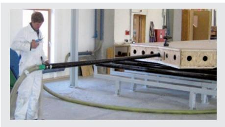
In modern timber construction buildings are erected in the minimum time with prefabricated elements. Wall and roof structures are manufactured in the factory, independent of the weather, and assembled at the building site.
