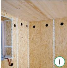
Depending on the degree of prefabrication, timber frame walls are either already filled with the cellulose insulation in the factory or filled onsite.
